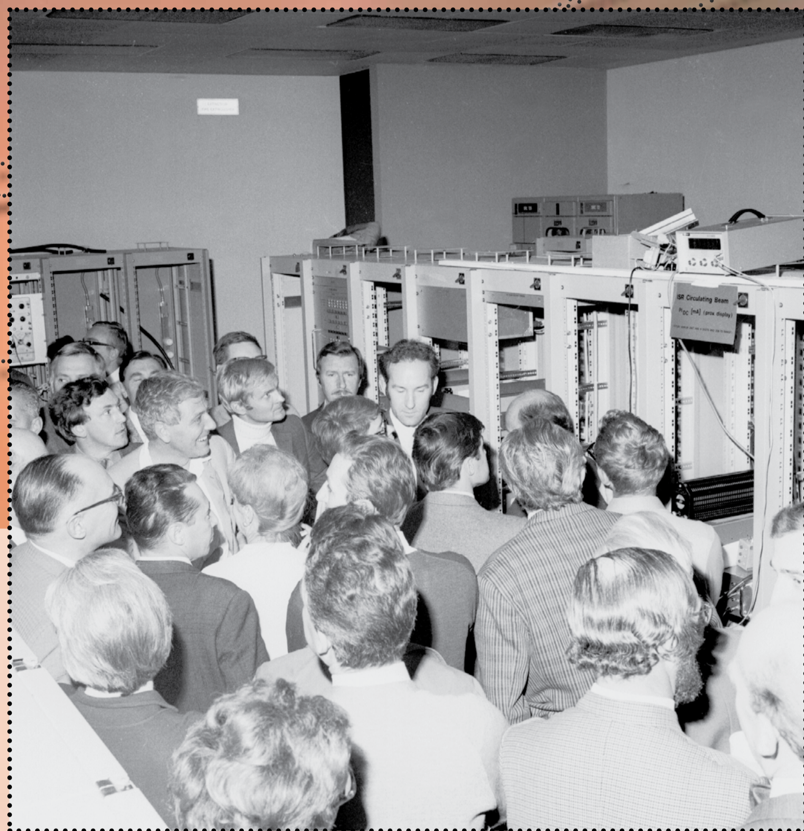
First injection tests into ISR Ring I. In the main control room, on the night of 29 October 1970, spectacular success was achieved with the first injection tests into Ring I. The focus of attention, top right, is a monitor which indicated the circulating beam current.
