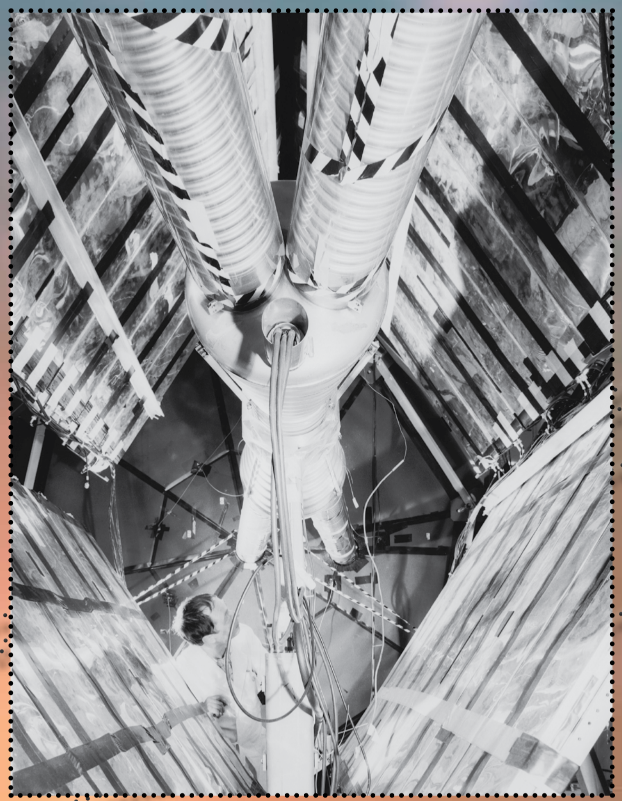
A vacuum chamber where the proton beams collide in the ISR, June 1973.
